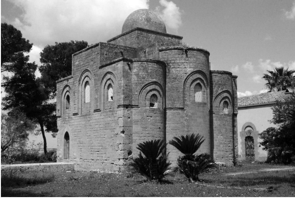
FIGURE 24.5. SS. Trinità, Delia, near Castelvetro, ca. 1150, exterior from southeast. Photo: Mark J. Johnson.
